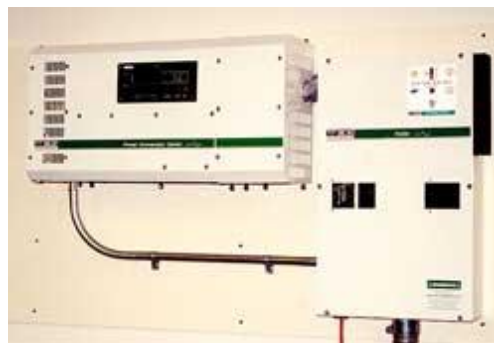
Trace 4 kW sine wave inverter and optional DC power center
