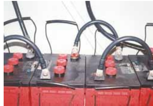
6-volt 350-amp-hour batteries with “Flag” terminals allow bolt-on type cable interconnects.
