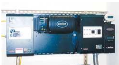
Outback 2 kW sine wave inverter including optional AC (left) and DC (right) power centers
