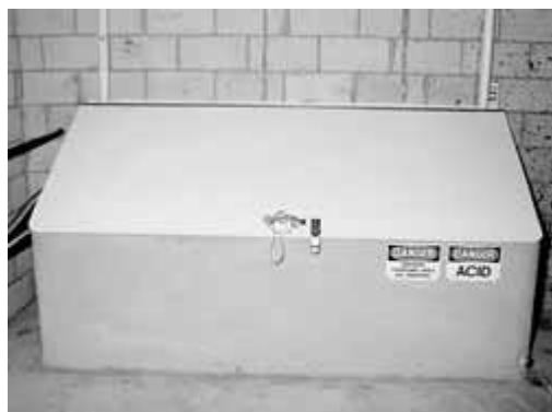
A well designed vented battery box. Note the warning signs and locked lid.
