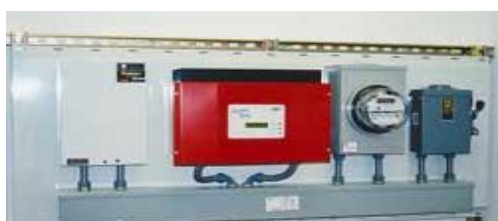
Sunny Boy grid-tie inverter, optional disconnects, and check meter
