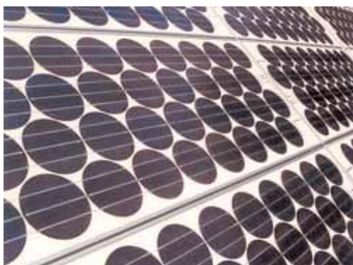
Round single-crystal Siemens (shell) modules. Note expansion space between module frames.
