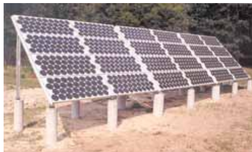
Siemens (shell) 100-watt modules ground-mounted with horizontal axis.
