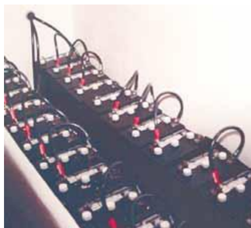
Interior view of the battery box showing the battery inter-connects and fuses.
