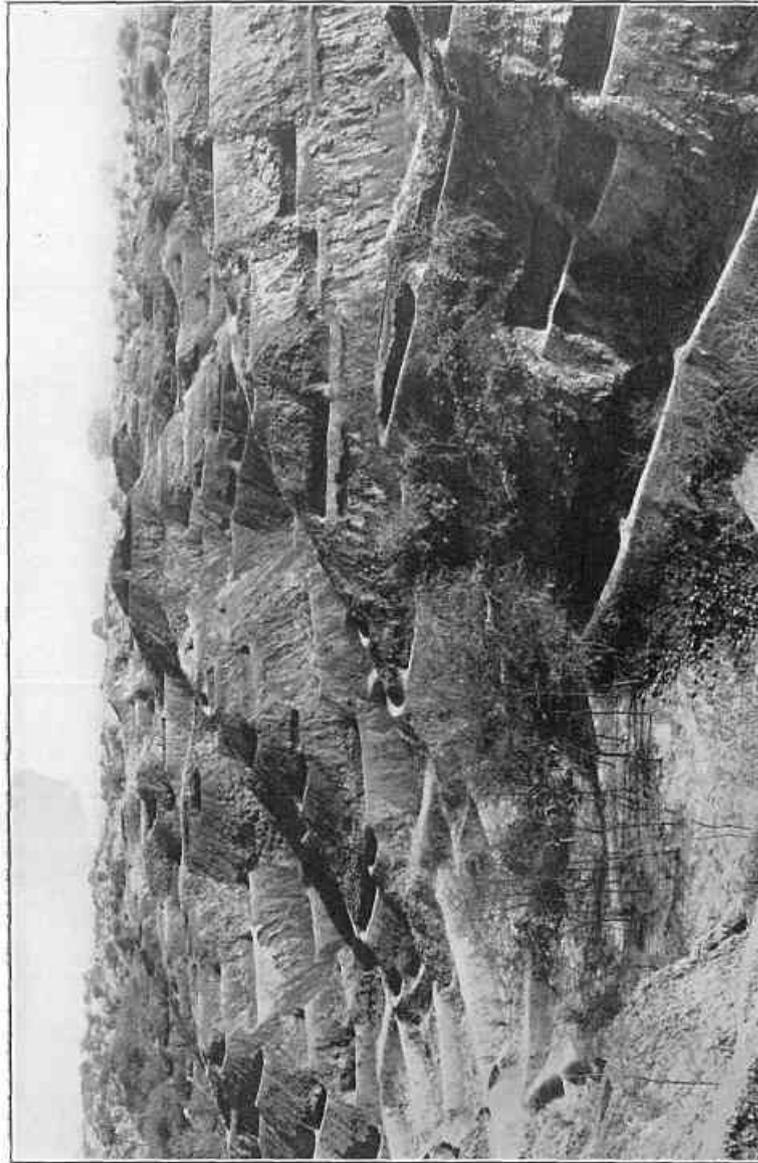
FIG. 113. Bare eroded lands on the upper Jumna were quickly reforested by digging these pits to catch rain water and irrigate the trees. Pits increased water penetration several fold, from 6 inches to 40 inches. Pits dug by famine relief funds.
