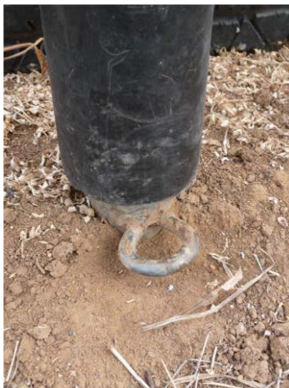
Eyebolt used to secure rope to ground posts
