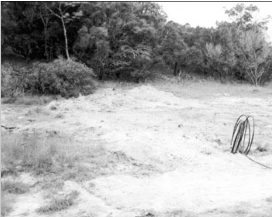
The site has been covered with earth trenched from the site. Notice the one-inch pipe; it has been connected to the nipples and is ready to be connected to the storage tank. Prehn seeds the construction site with native grass, and in a relatively short time the area will return to its original state, even much improved.
