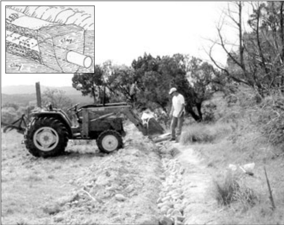
Covering the pipe with gravel.
