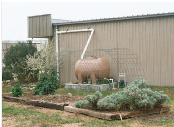
Rainwater captured from the 1,500-square-foot roof of the Walker County Extension office is stored in a 550-gallon polypropylene tank, a type readily available at ranch supply retailers. The 10-gallon flush diverter is the vertical standpipe visible to the left of the tank. Captured rainwater irrigates an adjacent Master Gardener demonstration garden, foreground.
