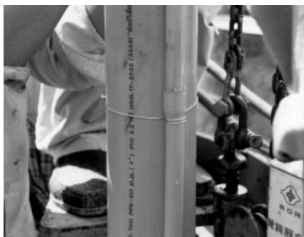
Figure 7.17 Use of small diameter pipe as centralisers
