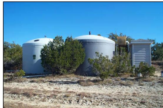
Figure 2-5. Two 10,000-gallon fiberglass tanks
