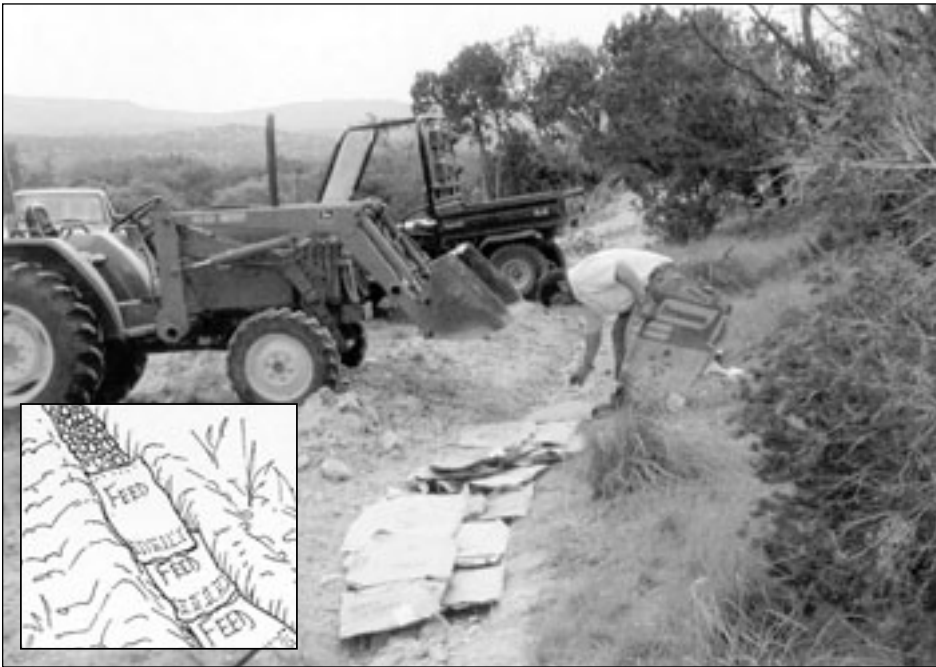
Prehn places sacks on top of the gravel. It's not imperative to use sacks, any pipe covering will do.
