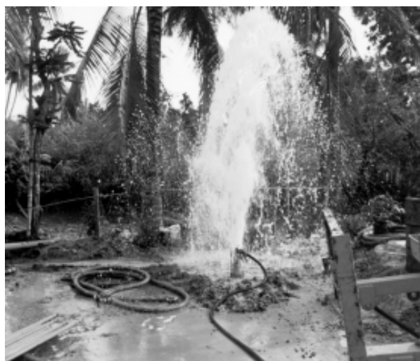
Figure 7.12 Final stages of developing with compressed air
