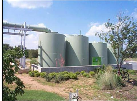
The H-E-B at the corner of Brodie Lane and William Cannon Blvd. in south central Austin irrigates an adjacent landscape of water-thrifty plants with rainwater stored in four painted steel tanks totaling 28,000 gallons. A 24-inch-diameter pipe conveys water from the roof to the tanks.
