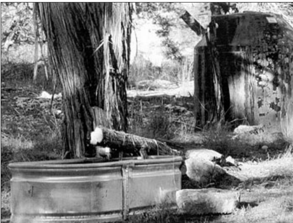
The storage tank for Site Four, with overflow on the tank and the water trough. Site Four produces about 600 gallons a day.
