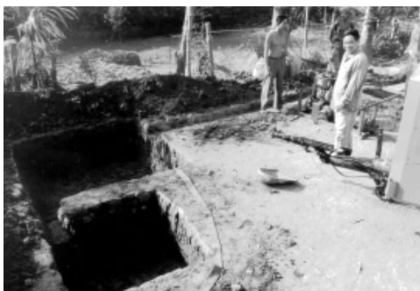
Figure 2.5 Well proportioned mud pits ready for filling
