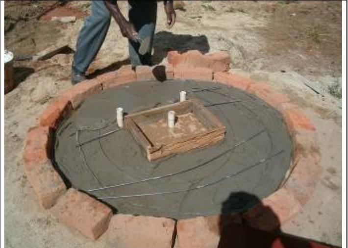
*Some reinforcement bars 6 mm plus wire should be placed. Not yet completed at the picture.*
