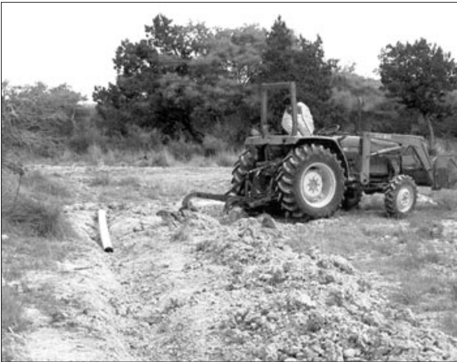
Site Four under construction. Prehn uses a tractor to dig the trench for the perforated pipe.
