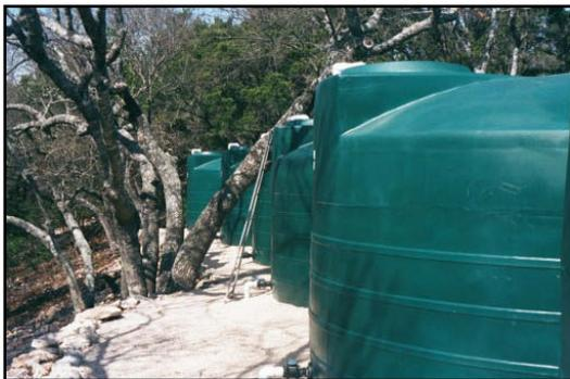
Figure 2-6. Low-profile 5,000-gallon polypropylene tanks
