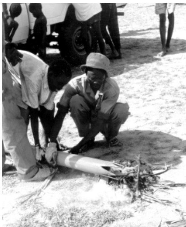
Figure 7.2 Heating up pipe end to form points
