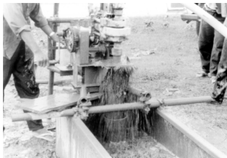
Figure 3.2 Drilling with compressed air – having "struck" water
