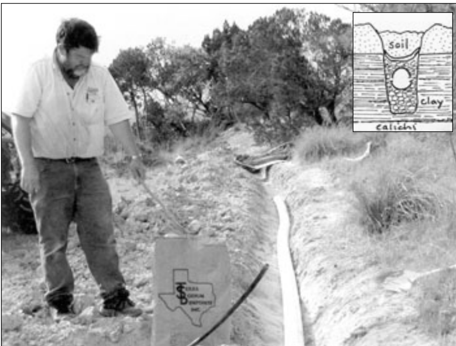
Prehn installs the pipe. Bentonite clay lines the trench.
