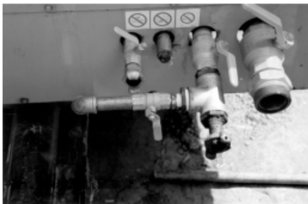
Figure 7.11 Air development manifold – Allowing discharge to atmosphere
